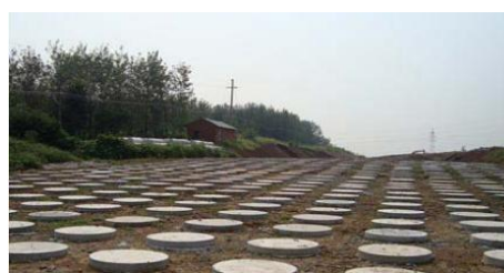
Fig.1 Soft Foundation Treated by CFG Piles
